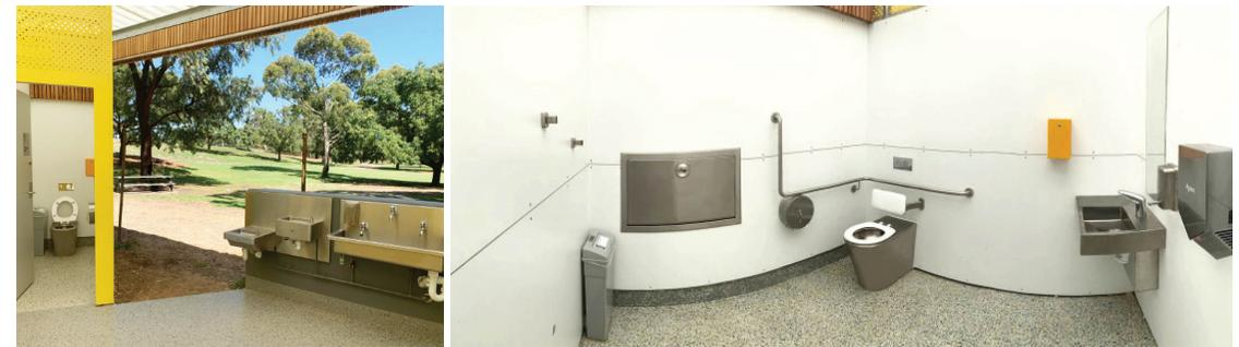
(L-R): Changing Places Facility and Public Amenities Block Facade, View of Britex Wall Mounted Hand Wash Trough and Wall Mounted Double Dado Drinking Fountain with Accessible End, View of Ambulant Toilet Cubicle with Britex Vandal Resistant Centurion Ambulant Pan fitted with Vandal Resistant White Toilet Seat, Hand Wash Trough and Drinking Fountain, View of a complete accessible fit out with Britex Toilet Pan and Accessible Bellagio Basin with integrated shelf.
