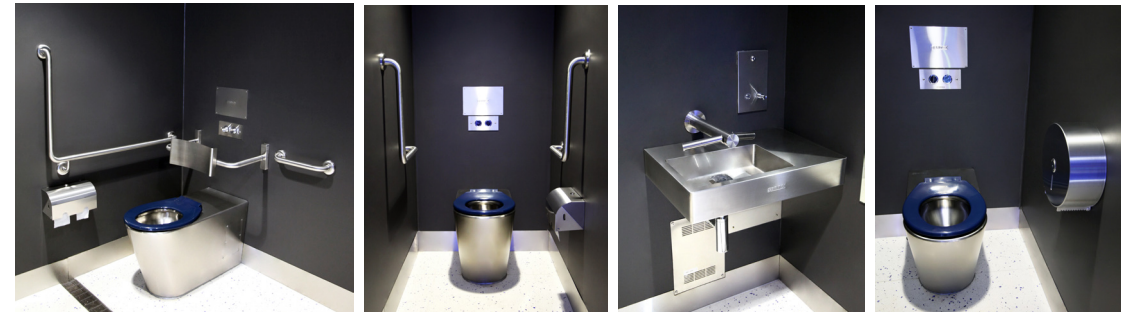
(L-R) Britex S.S. In Wall Cistern with Raised Accessible Buttons, Britex S.S. Centurion Disabled Toilet Pan with Navy Vandal Resistant Closed Front Toilet Seat, Britex S.S. Adjustable Straight Arm Backrest with Vandal Proof Pad, Britex S.S. In Wall Cistern with Raised Accessible Buttons, Britex S.S. Centurion Ambulant Toilet Pan with Navy Vandal Resistant Closed Front Toilet Seat, Britex S.S. Accessible Bellagio Hand Wash Basin with Integrated Side Shelf, Britex S.S. In Wall Cistern with Standard Buttons, Britex S.S. Centurion Toilet Pan with Navy Vandal Resistant Closed Front Toilet Seat.
