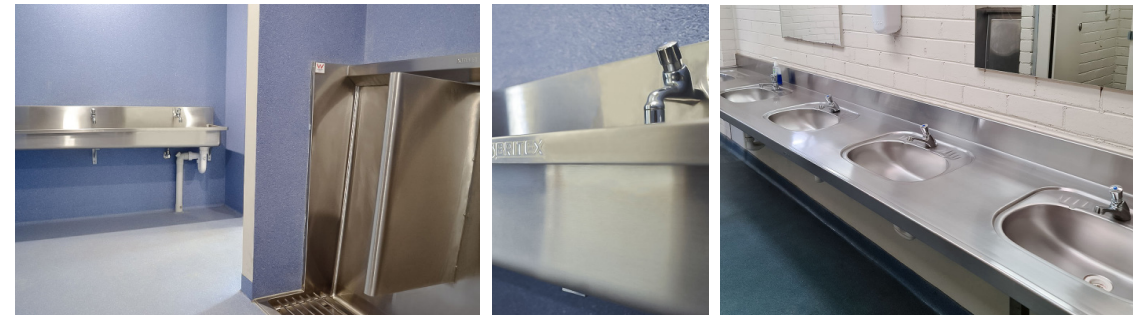
(L-R): Top - A view of Kambrya College, view of Britex Stainless Steel Sanistep Urinal with Urinal Privacy Panels, view of Britex Stainless Steel Preplumbed Hand Wash Trough, close up view of Britex Stainless Steel Preplumbed Hand Wash Trough with Wall Mounted Push Button Tap and view of Britex Stainless Steel Multi Vanity Hand Basin.
